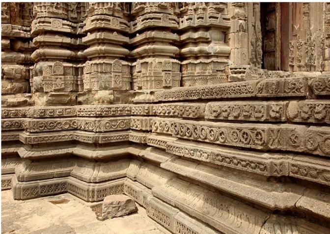
**Fig -8: Typical moulding plinths of Yadava temple**
